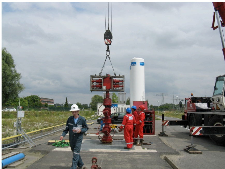
Observation well Ktzi200 during preparation of the lubricator system for the downhole seismic measurements (photo: courtesy of GFZ).
