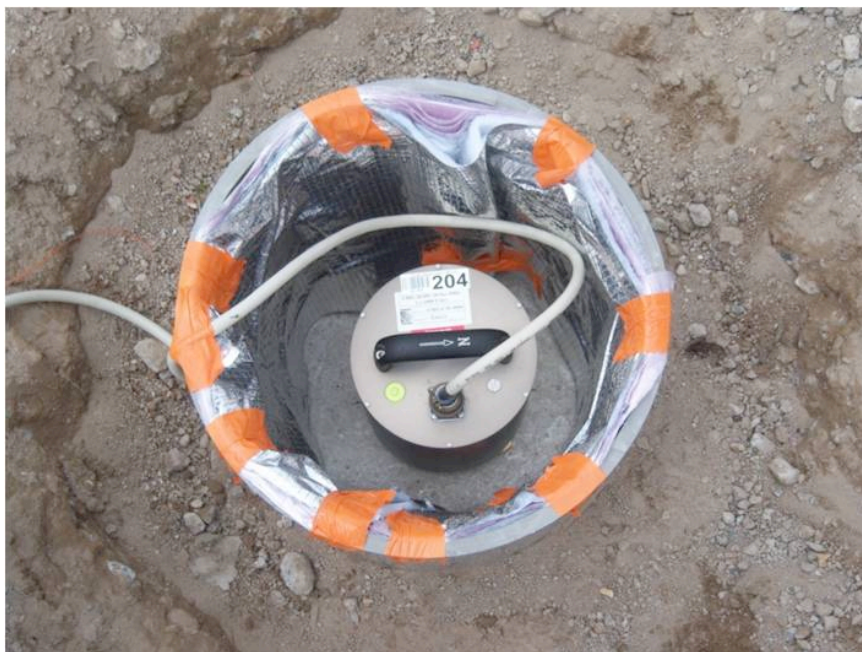
Buried broadband seismometer and isolation installation (photo: courtesy of BRGM).
