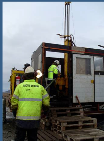
Drilling rig close to Longyearbyen
